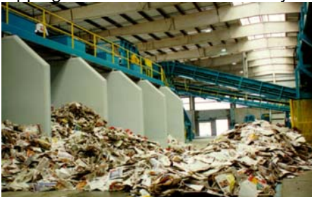
Once sorted, recyclable materials are moved via conveyor
