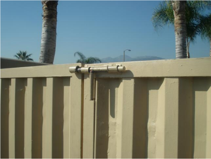
Close-up view of Gate Latch
